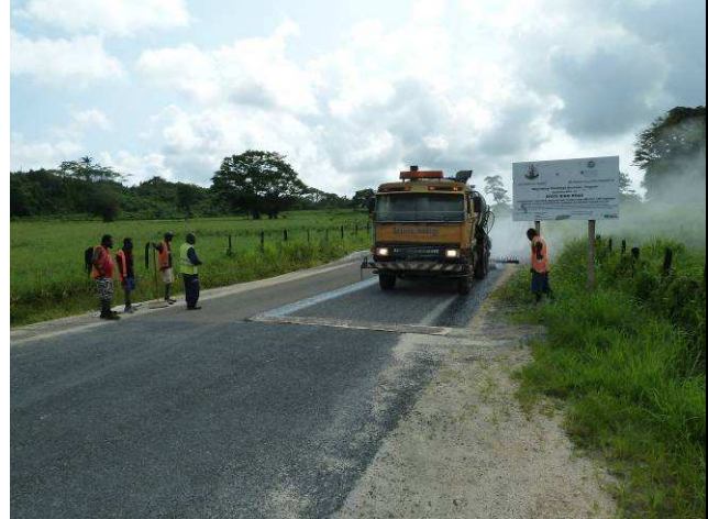
The sprayer approaches the end of the Project length on the last full width spray run.
