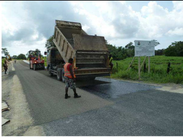
Spreading the sealing chip on the final spray run.
