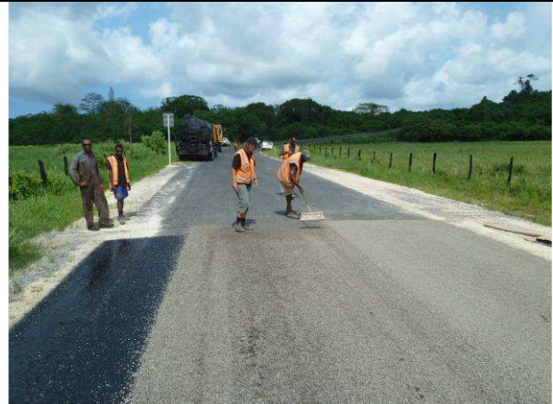
Tidying up. Sprayer operator Richard, Sealing Engineer Wendy Heynan and Joel Kalsal checking the last seal joint.
